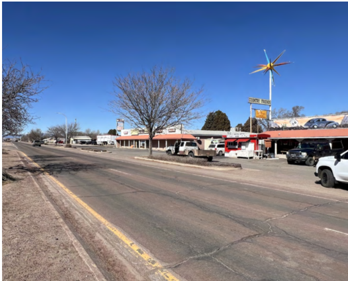
Route 66 Currently Lacks Pedestrian Facilities
