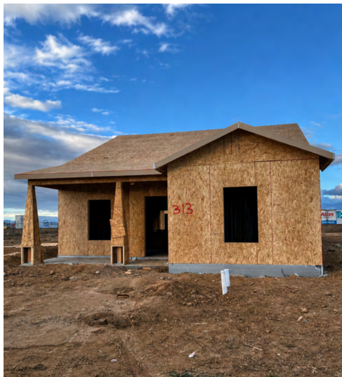
Construction of Single-Family Home in Moriarty
