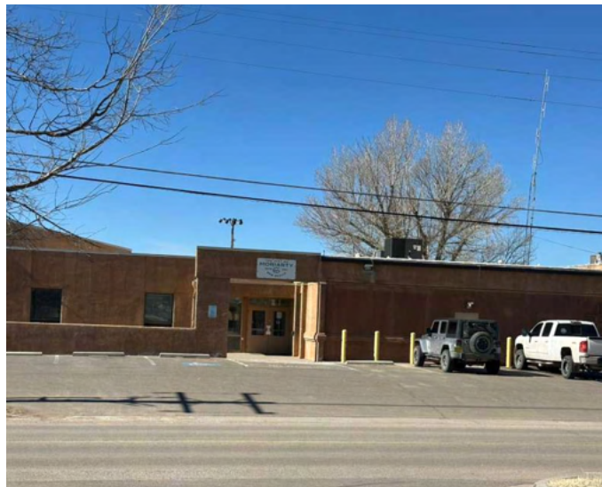
City of Moriarty City Hall
