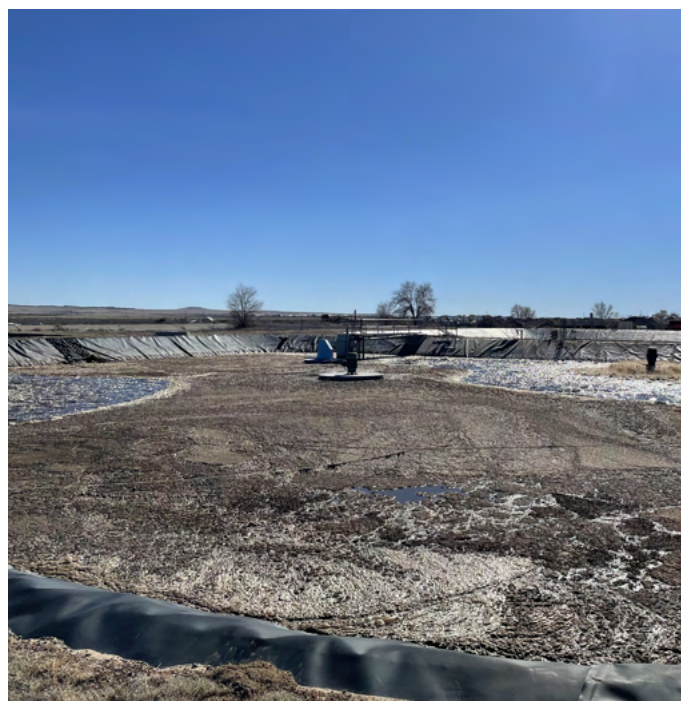
Wastewater Treatment Facility in Moriarty
