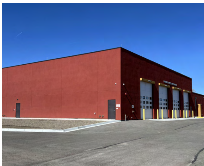
City of Moriarty Fire Department Station
